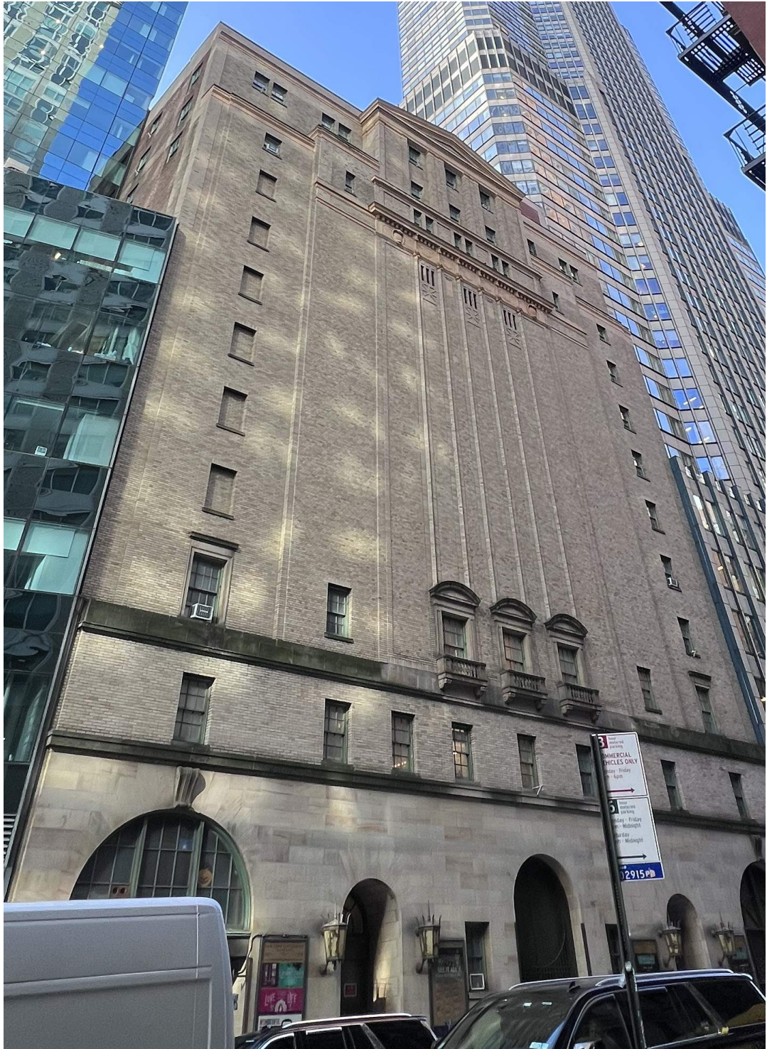
2. 56TH STREET : FRONT VIEW
