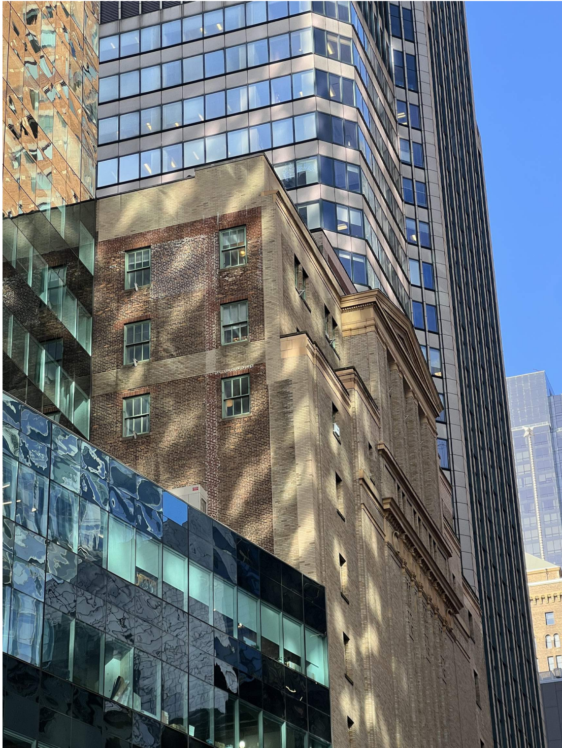
1. 56TH STREET - VIEW FROM NORTH EAST CORNER
