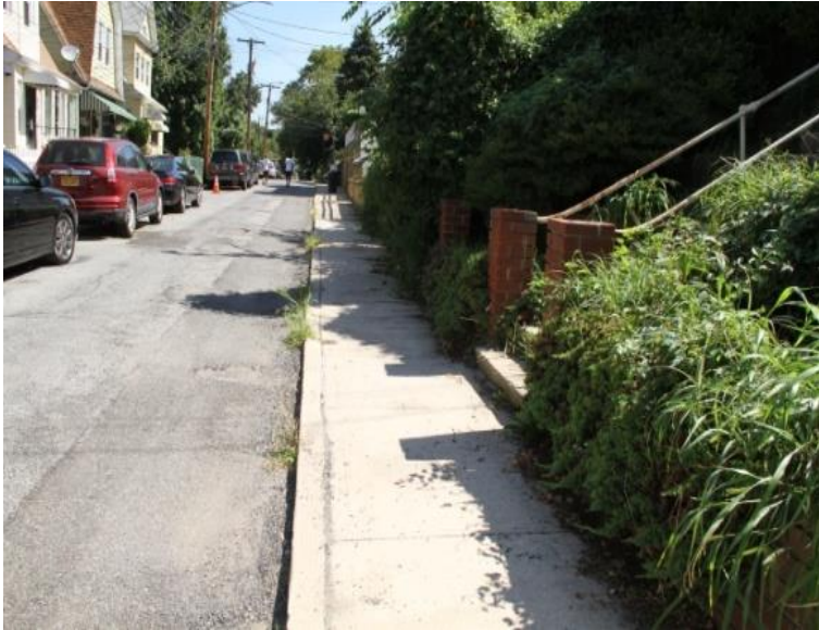
Picture 6: Existing Roadway and Southern Sidewalk I/F/O House No.46 (Photo taken looking towards York Avenue)
