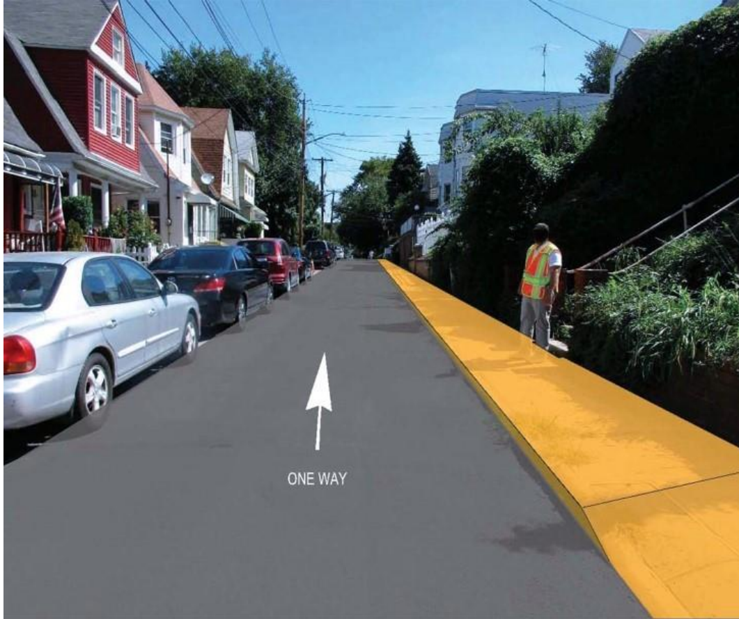
Van Buren Street Near Minerva Place Facing East
