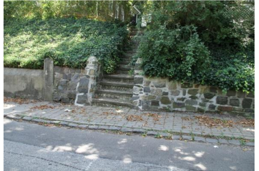
Picture 8: Existing Southern Sidewalk and Stairs for House No.14
