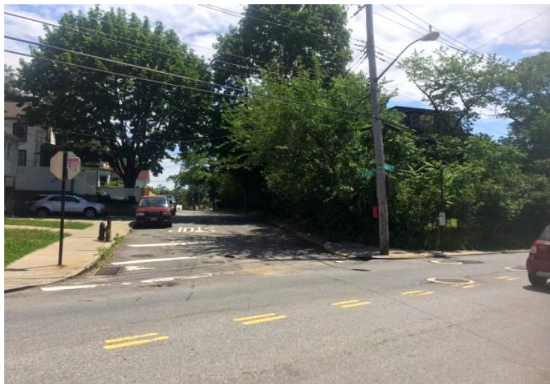
Picture 7: Existing Roadway and Sidewalk at the intersection of Alaska Street & Richmond Terrace (Photo taken looking towards Alaska Street)
