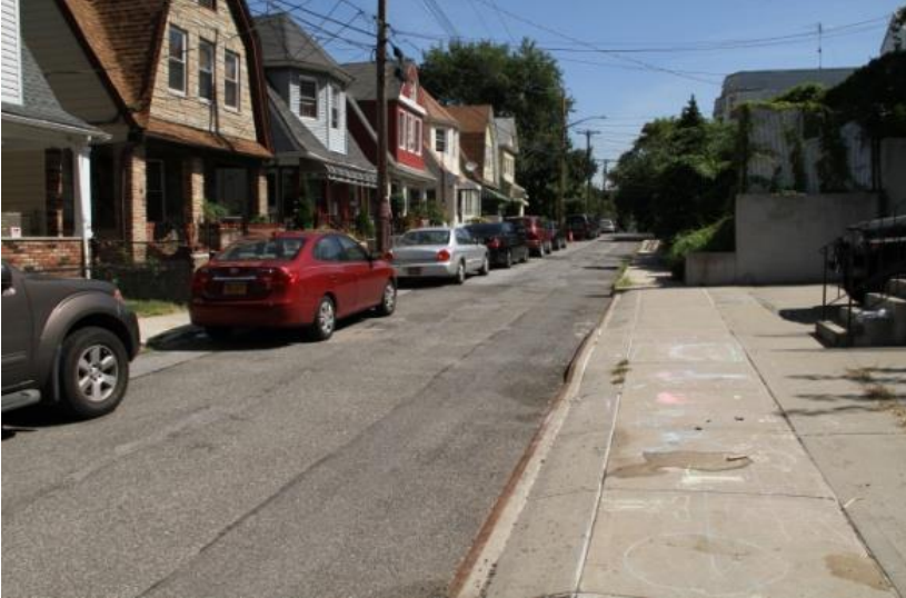
Picture 3: Existing Roadway and Southern Sidewalk I/F/O Lots No.29 and No.27 (Photo taken looking towards York Avenue)
