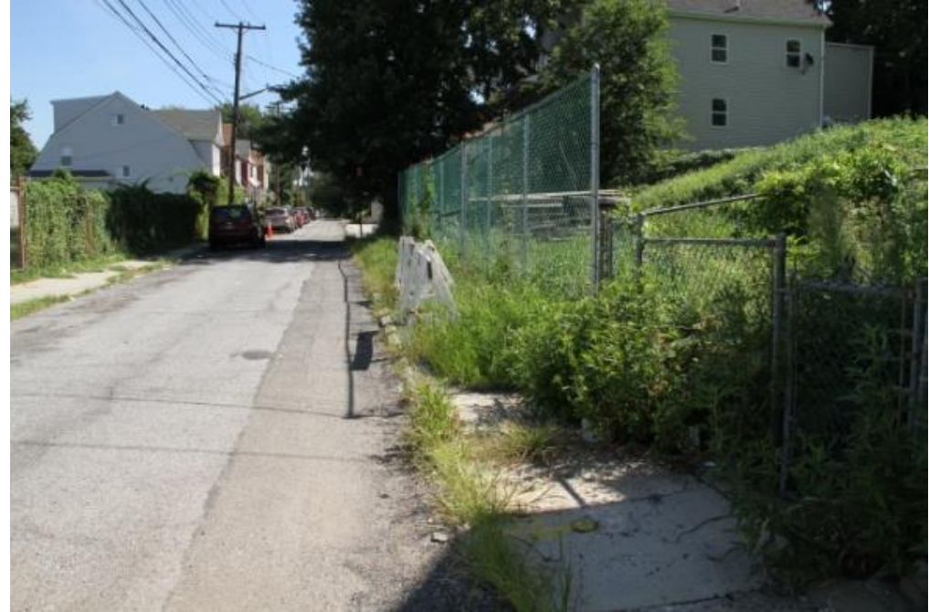
Picture 2: Existing Roadway and Southern Sidewalk I/F/O Lots No.36 and No.34 (Photo taken looking towards York Avenue)
