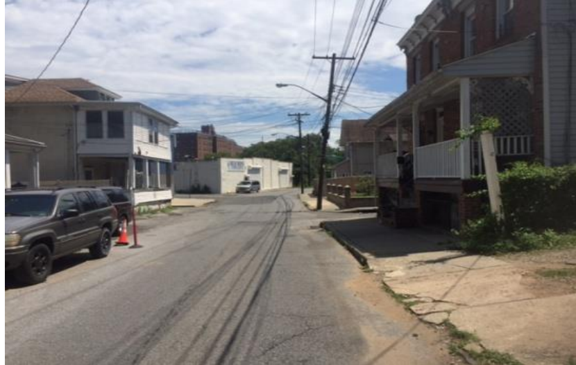
Picture 5: Existing Roadway and Western Sidewalk I/F/O House No.52 and No.54 (Photo taken looking towards Woodruff Lane)
