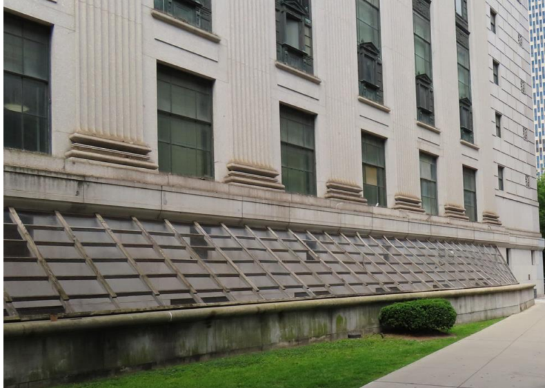
Existing temporary enclosure at Worth Street Window Well
