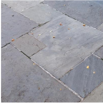
Bluestone Pavement to match existing
