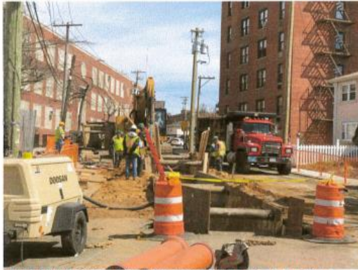
SANITARY SEWER PLACEMENT LOCATED AT BRIAR PLACE ALONG BROOKHAVEN AVENUE & COLLIER AVENUE
