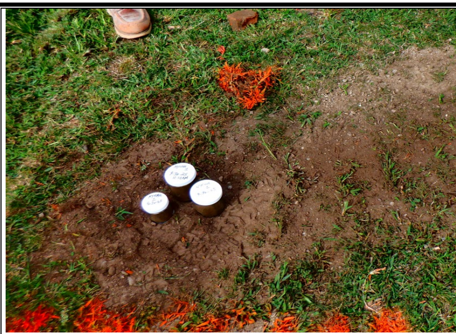
Soil boring NYCHA 1, collected 9/30/25
