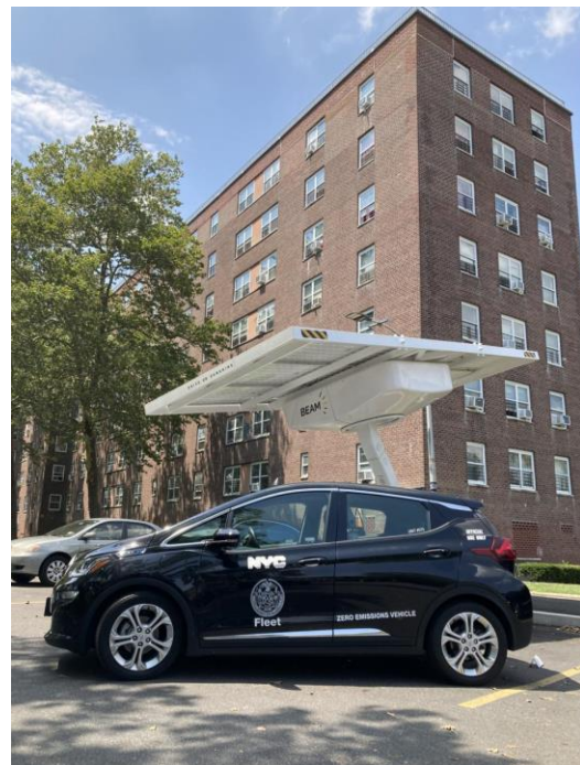
DCAS solar carport and shared Bolt at Sotomayor Houses in the Bronx.
