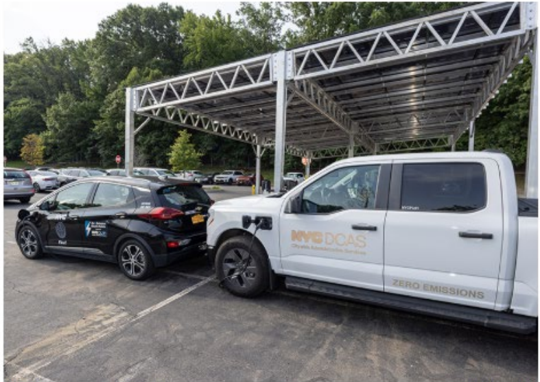
Pictured Above: DCAS electric vehicles parked in front of the solar canopy at Michael J. Petrides School, Staten Island
