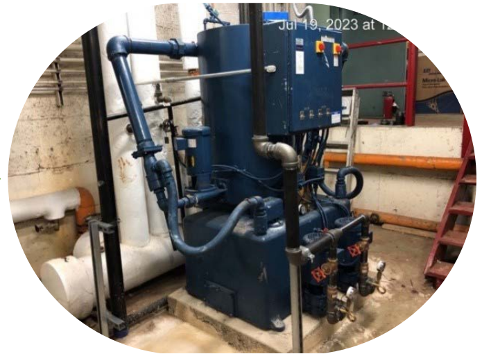
After - A replaced vacuum condensate unit
