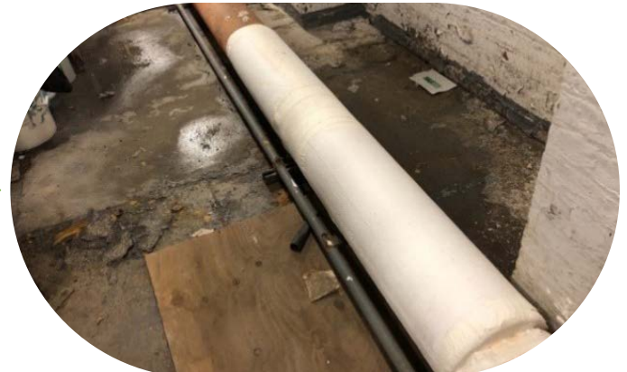
After - An insulated pipe
