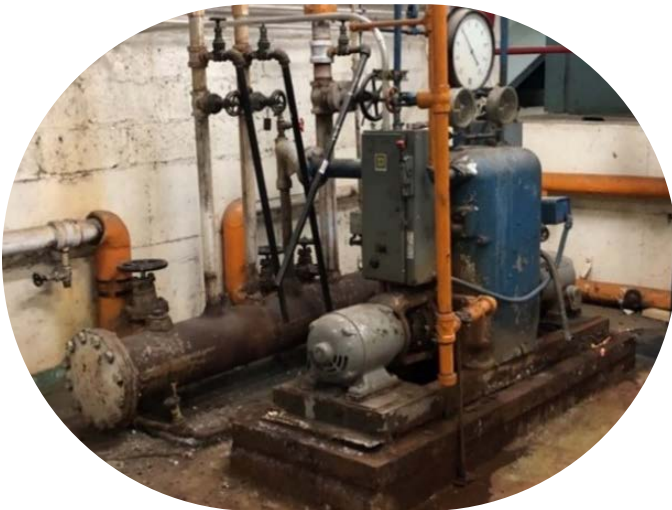
Before - A failed vacuum condensate unit
