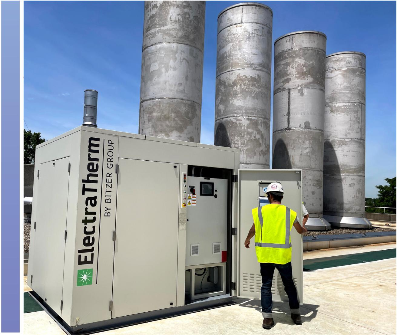
DCAS staff inspecting a recently installed new technology project as part of DCAS's Innovative Demonstrations for Energy Adaptability (IDEA) program. This installation captures waste heat and generates electricity.
