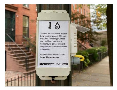
[FIGURE 16 **A**] A temperature sensor installed in Brooklyn for a rapid IoT pilot with MOR.
