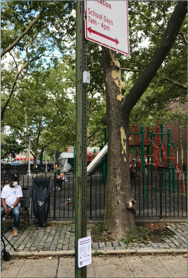
[FIGURE 01 ◀ ] Temperature/Humidity sensor installed in Brownsville, Brooklyn. Photo: NYC CTO
