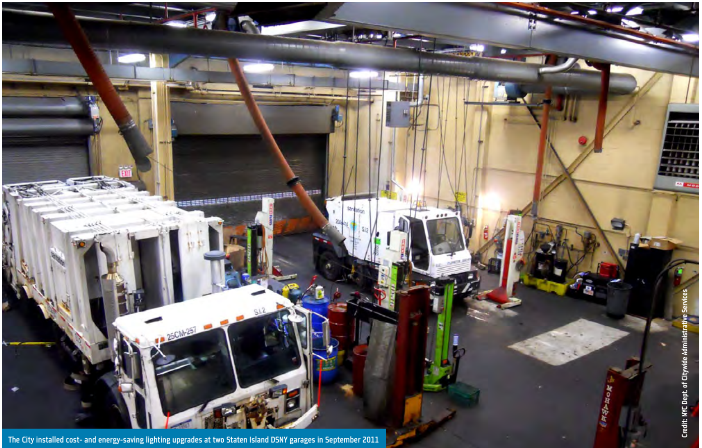
The City installed cost- and energy-saving lighting upgrades at two Staten Island D5NY garages in September 2011
