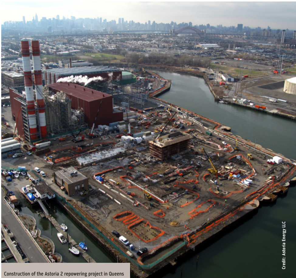
Construction of the Astoria 2 repowering project in Queens
