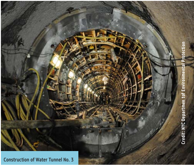
Construction of Water Tunnel No. 3
