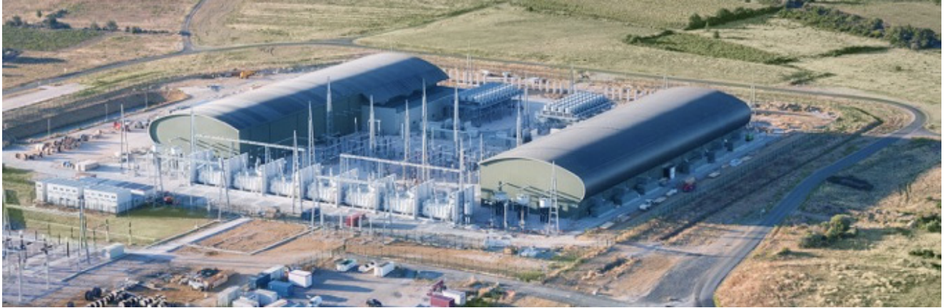
Figure 4. A Modular-Multilevel-Converter station, similar to what could be built on Rikers Island. xlix
