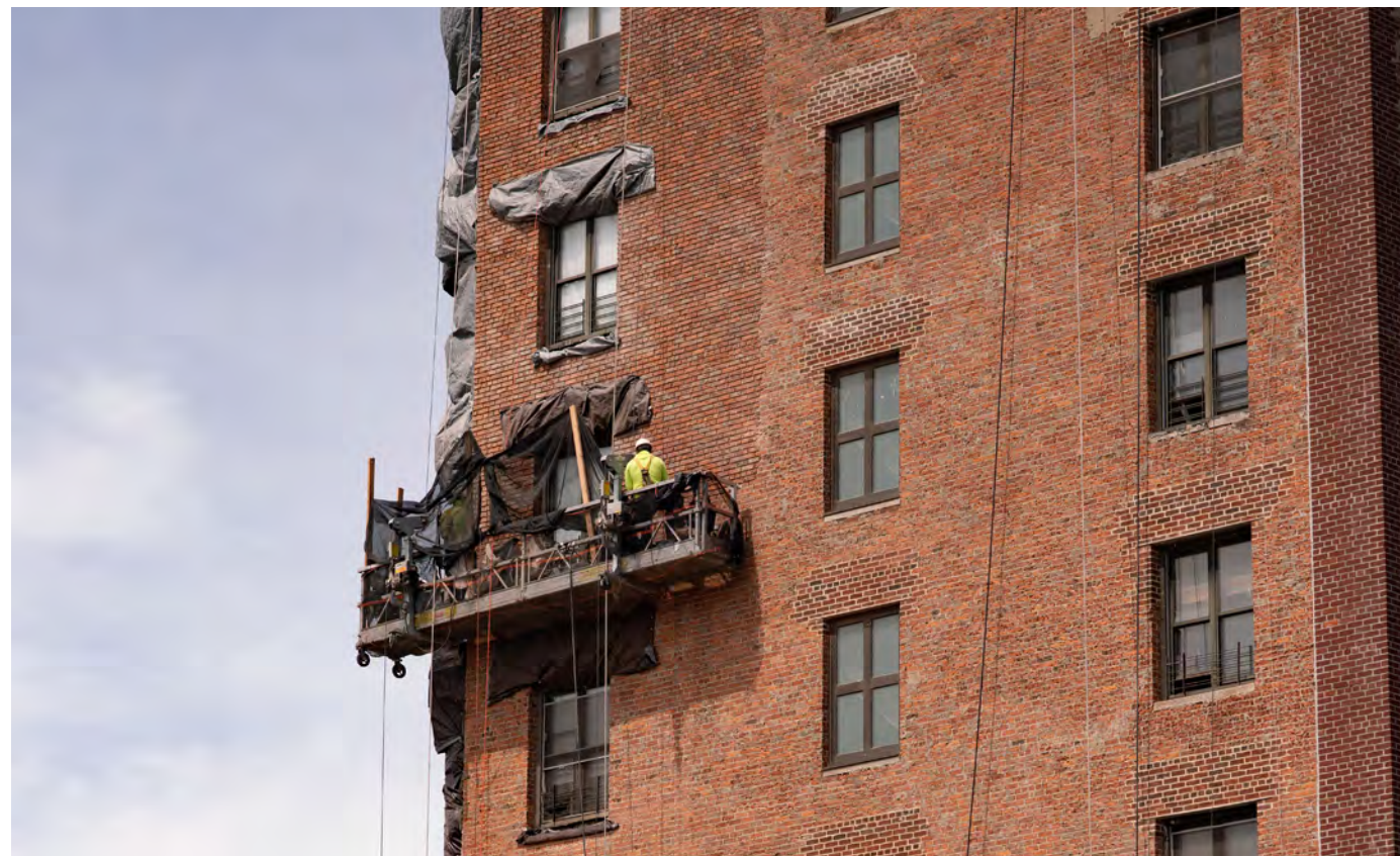
Building envelope improvements are an important retrofit solution to reduce heat and energy loss in buildings, cut GHG emissions, and enhance occupant comfort. Source: MOCEJ
