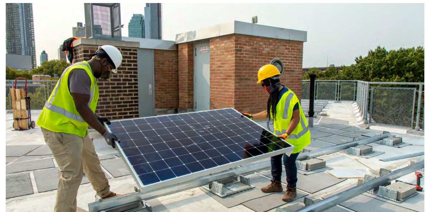
Solar panel installation on the roof of Queensbridge Houses. Source: NYCHA
