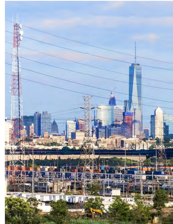
Grid transmission infrastructure. Source: Adobe Stock.
