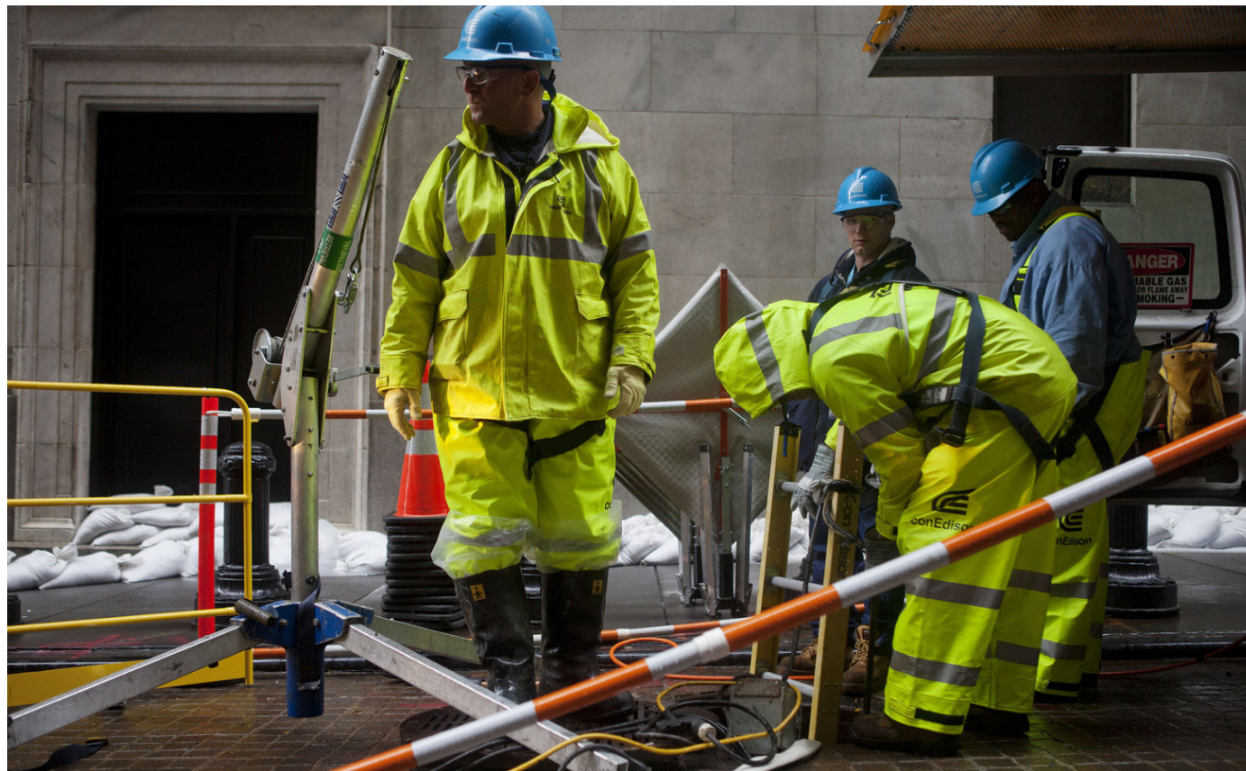
Utility repair in progress, Manhattan. Source: MOCEJ
