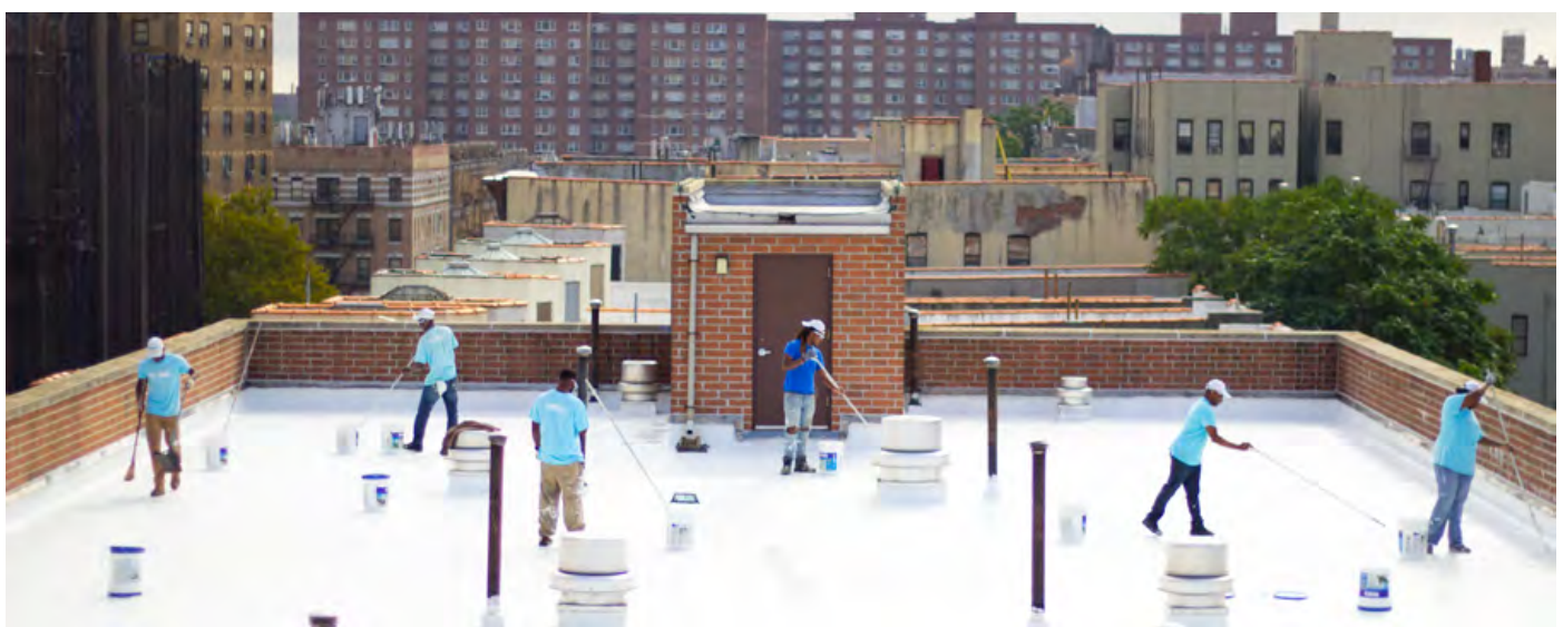
VOLUNTEERS WITH SUSTAINABLE SOUTH BRONX HELP PAINT A ROOFTOP WHITE AT AN NYC COOLROOFS PROJECT SITE.
