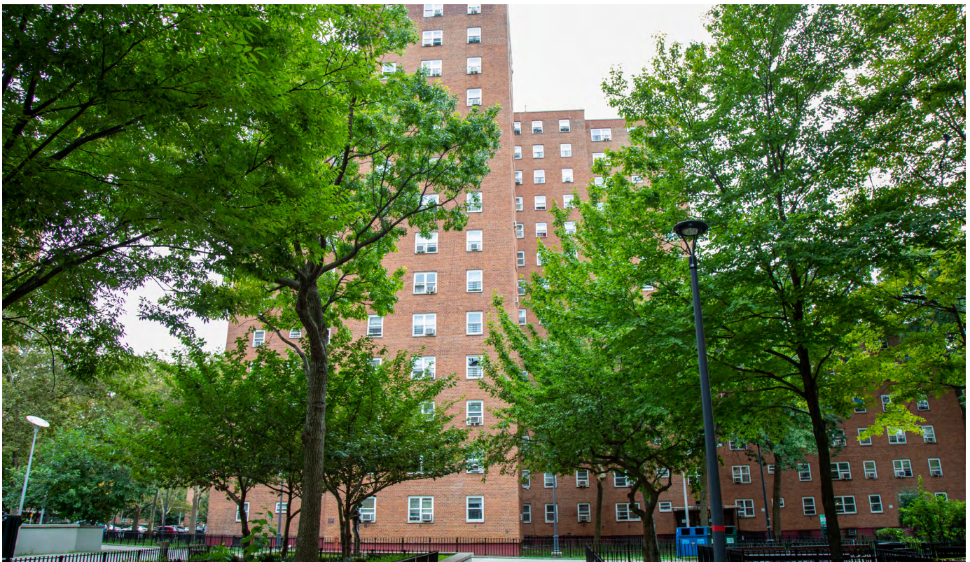
Canopy at Johnson Houses, Manhattan NYCHA
