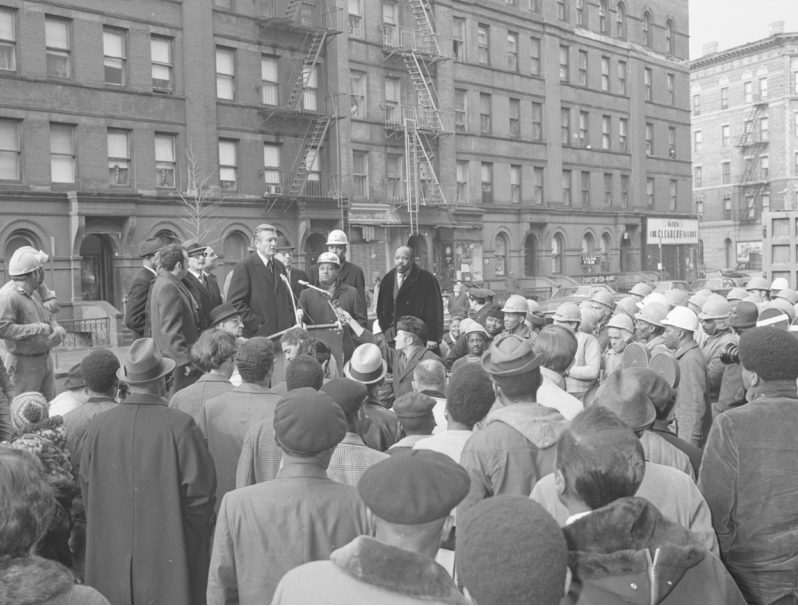
Mayor Lindsay, community members and construction workers at St. Nicholas Avenue and West 118th to announce the rehabilitation of the Garden Court apartment building.
