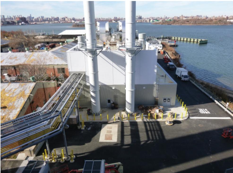
CHP uses waste heat from the electricity-generating process to produce steam for heating, which makes such systems more efficient than boilers. The new CHP facility underway at Rikers Island will include two 7.5 megawatt (MW) combustion turbines with heat recovery steam generators, for a total of 15 MW installed capacity. The facility will generate nearly all of the electricity and steam needed to serve Rikers Island, and is projected to save the City nearly \$7 million annually.
