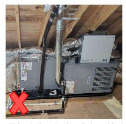
Units shall not be installed outside the thermal envelope. Where condition is observed, Applicant must be notified to recommend remedy
