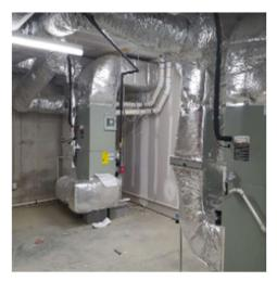
Verify that all ducts are sealed & fully encased with insulation as specified
