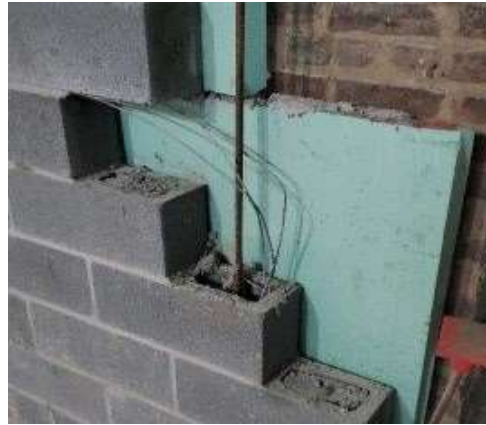
XPS installed on wall with no label visible requires close up measurement & spec.
