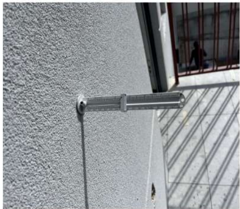
Gauge should be used to verify full depth of rigid insulation measured to substrate
