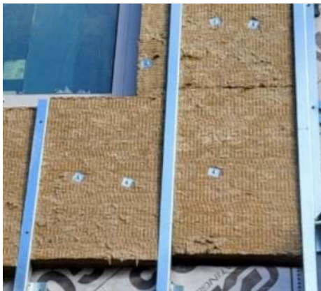
Mineral wool on exterior should be secured properly within full cavity of girts
