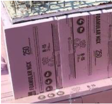
XPS installed without gaps that has clearly visible labeling is acceptable
