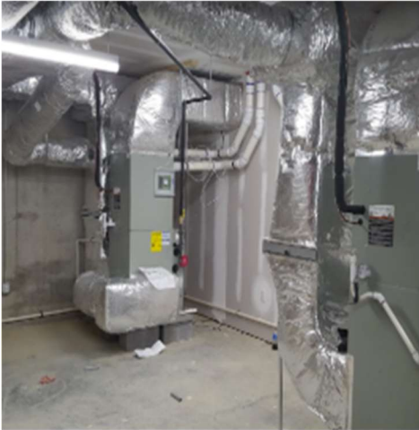
Verify that all ducts are sealed & fully encased with insulation as specified
