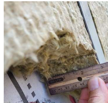
Mineral wool or unfaced batt installed to face of framing requires measurement
