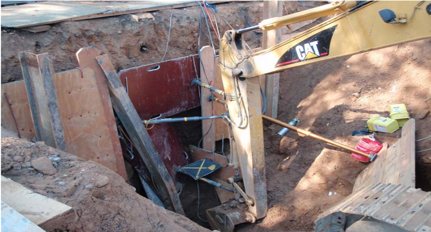
Example: Improper means and methods/sequence for SOE installation – excavation performed without first installing lagging
