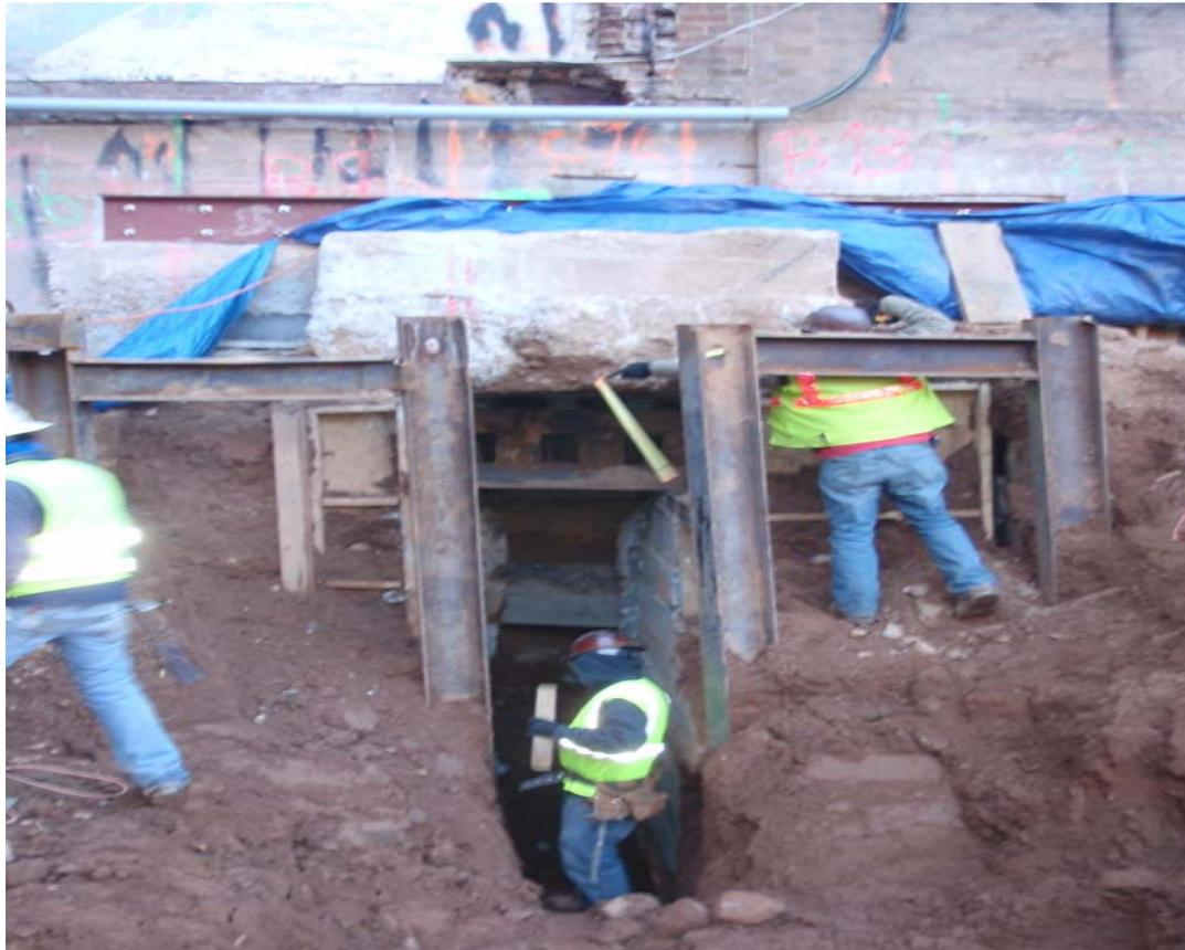
Proper design and construction: 10 foot by 10 foot footing of a three-story building column was underpinned without causing any damage
