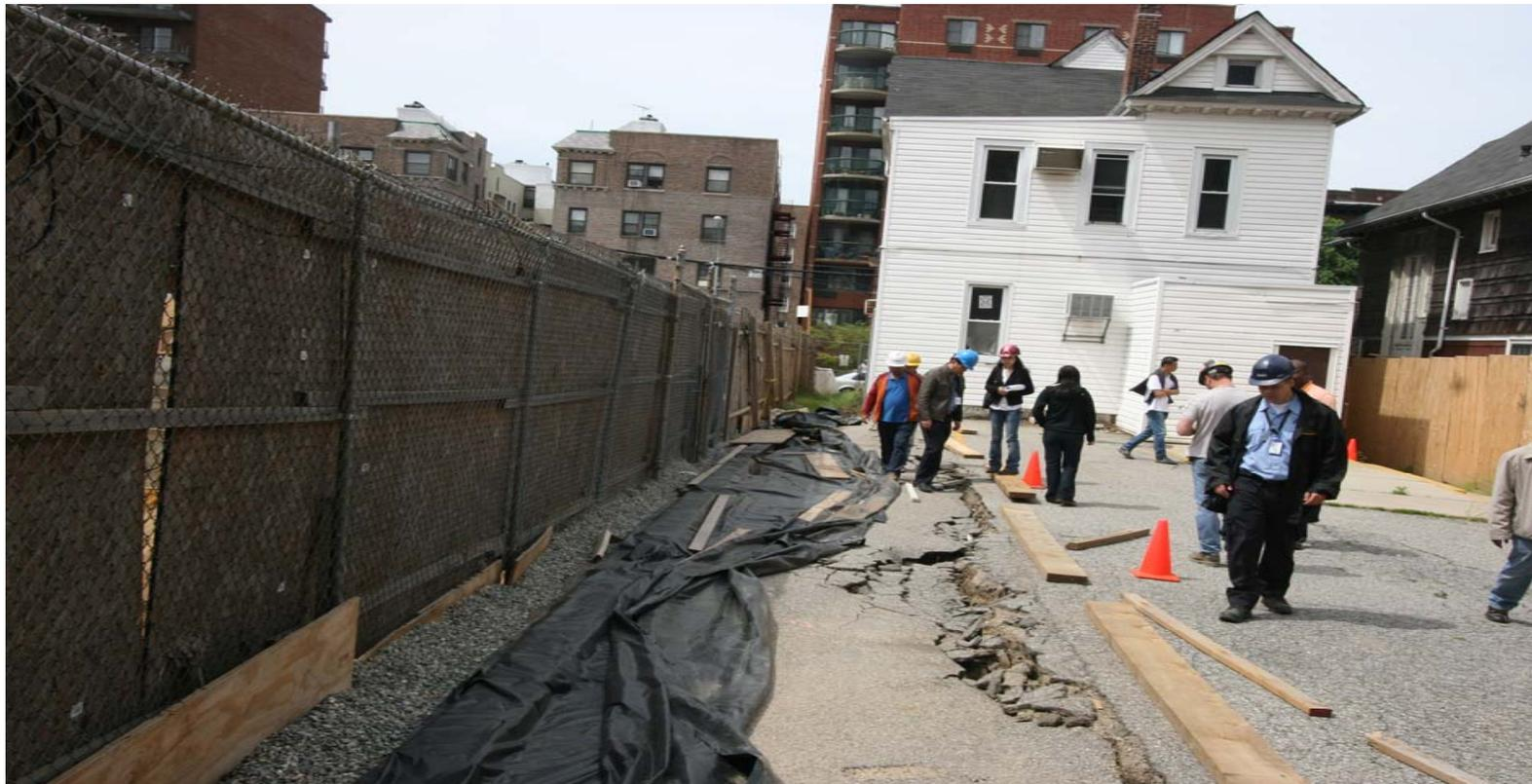
Example: Tension cracks visible at top of the supported soil by SOE shown in the last slide: improperly designed SOE.
