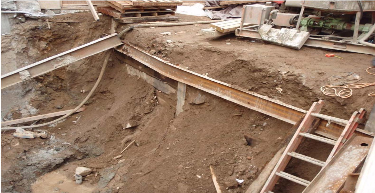
Example: No lagging provided; steel placed without any connections
