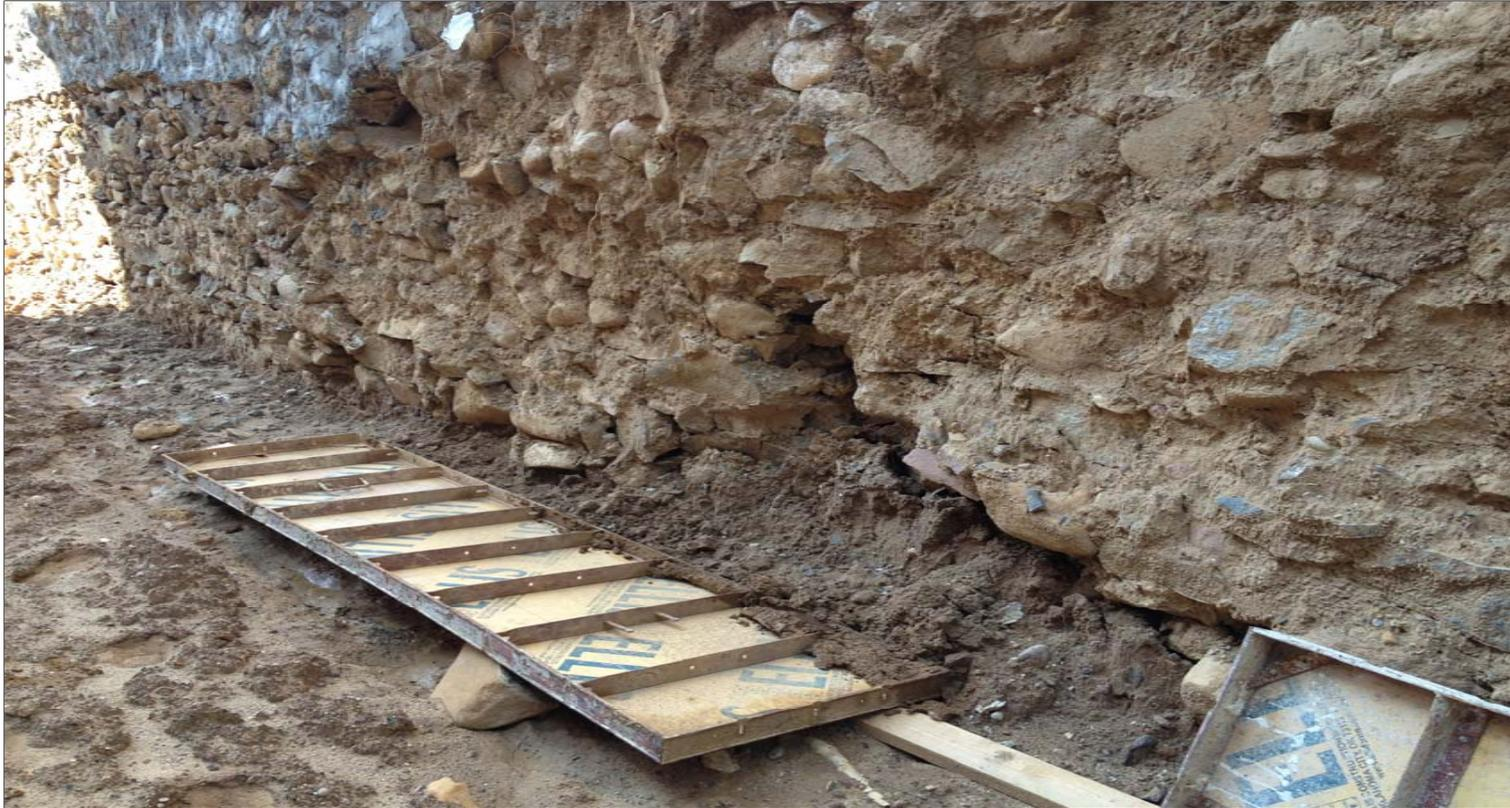
12-foot high vertical shear cut; no SOE or angle of repose visible
