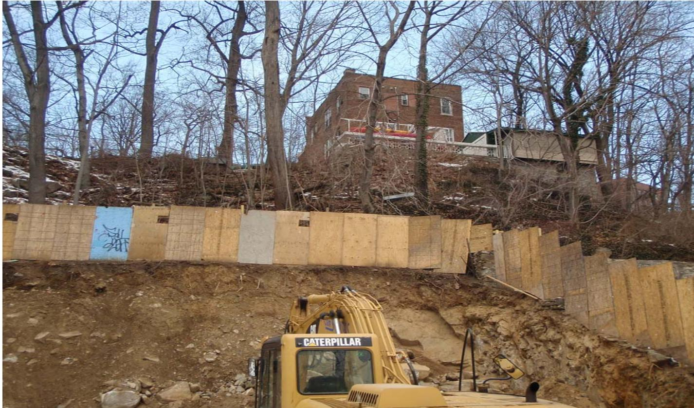
Example: 15-foot high shear cut; no SOE or angle of repose visible
