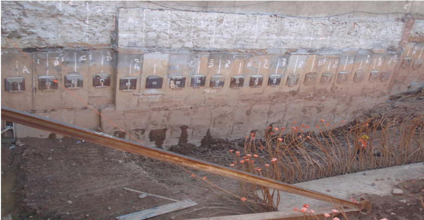
Multi-tier underpinning works if properly designed, sequenced and monitored.
