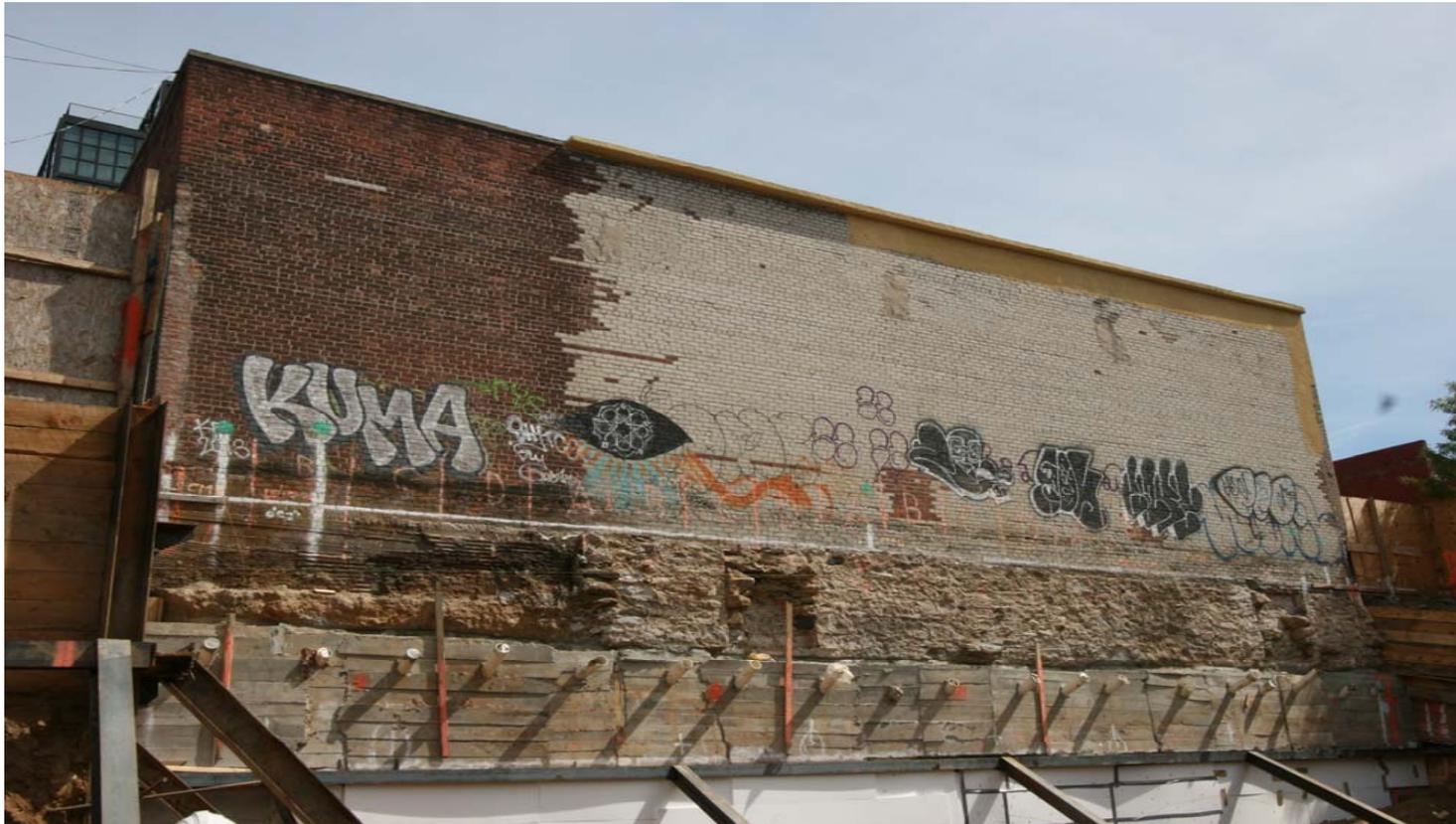
Example: Pins too long and installed originally – without bracing
