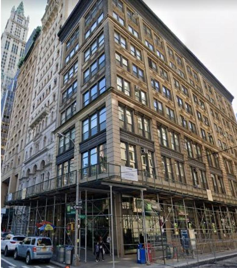
Mesh parapet for required for sheds installed under 2022 Code:
