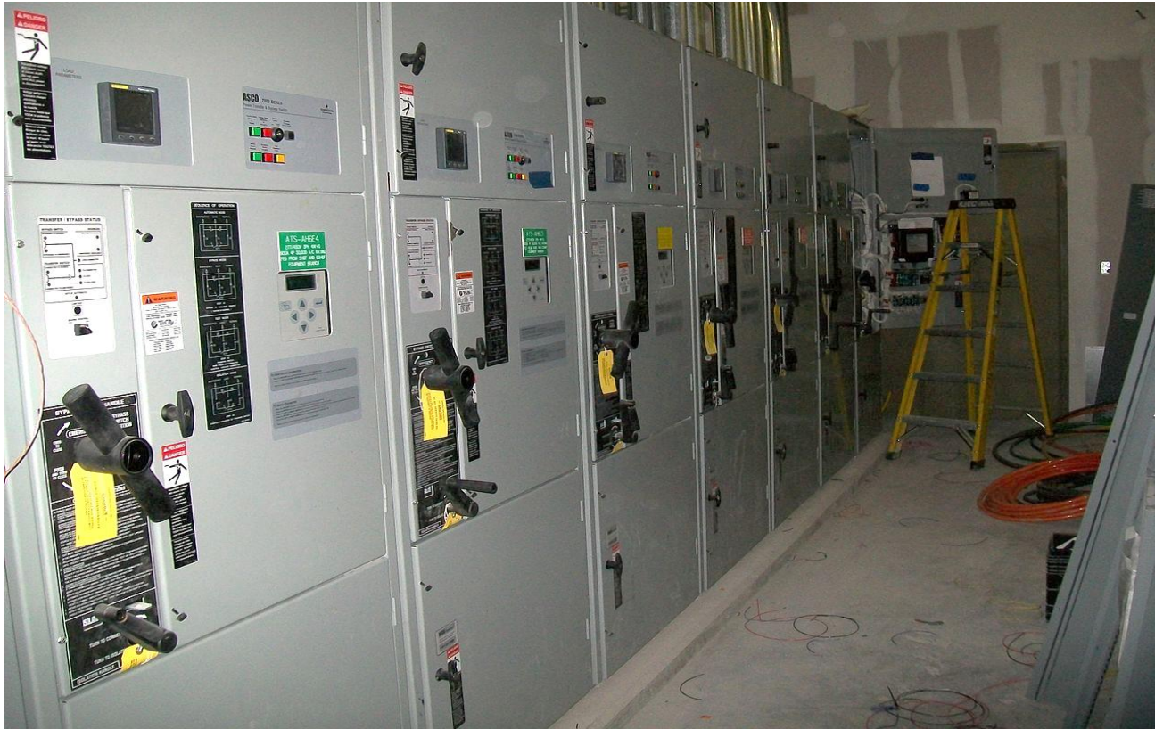
Figure 2702.1.7.1-4: Dedicated ATS Room for Emergency and Required Standby Systems
