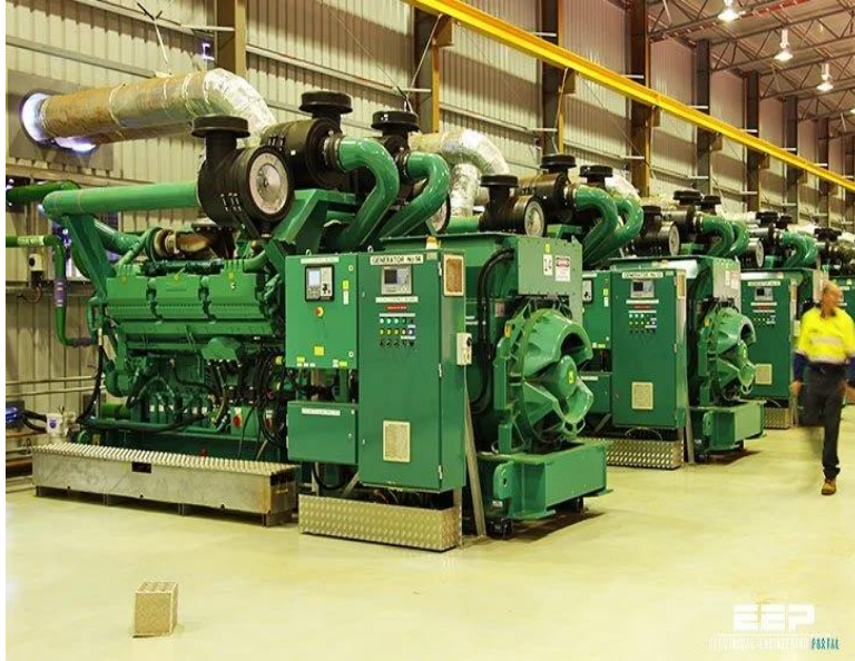
Figure 2702.1.2-3: Multiple generators sharing a common room
