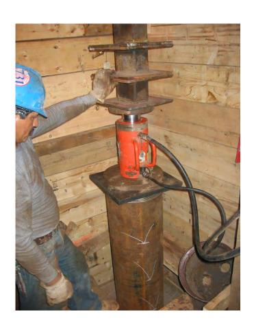
Where the method of support includes deep foundation systems such as pile supported underpinning or tie anchors, several requirements shall be met related to:
