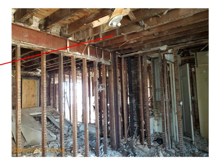
Open wood joists/missing firestopping
