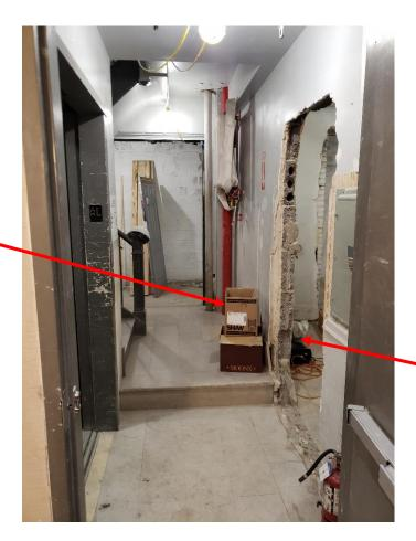
Fire-rated corridor construction is compromised. Temporary protection or Fire Watch is required.
