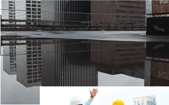
Source: Inadequate roof drainage
