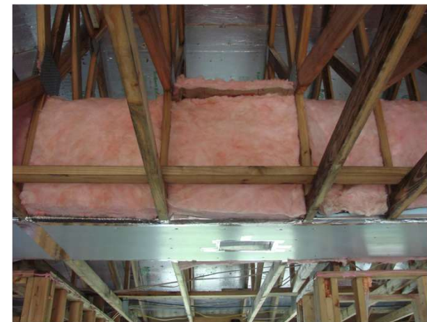
Figure MS-28-b Finished raised ceiling duct chase
