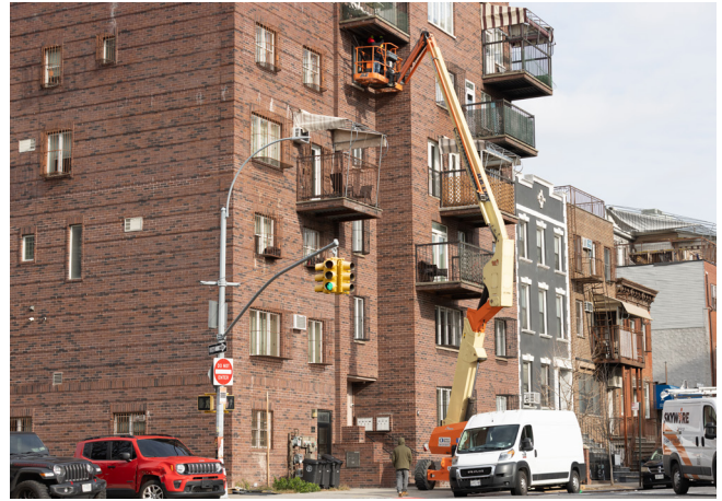
A boom lift is used to gain access to a façade in NYC.
