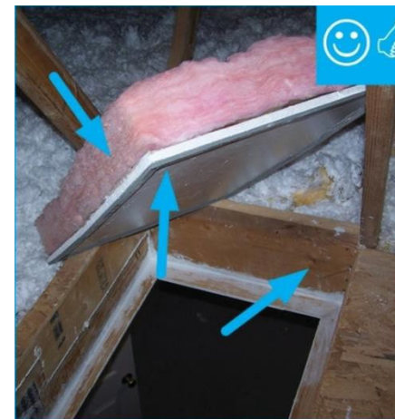
Figure BE-21-b Access Hatch Properly Insulated
