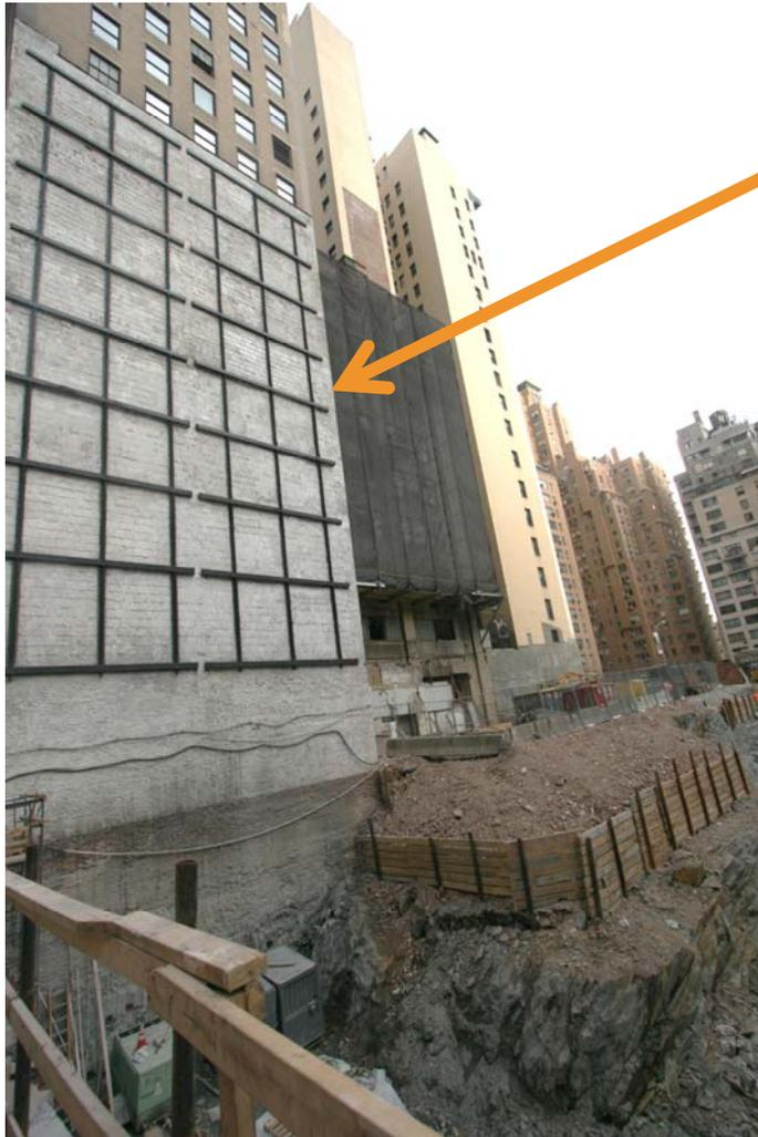
Lot-line façade of existing High-rise that is adjacent to the construction site = **fragile condition**
