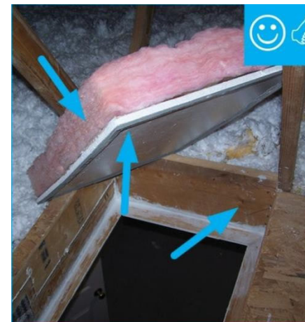
Figure BE-21-b Access Hatch Properly Insulated
