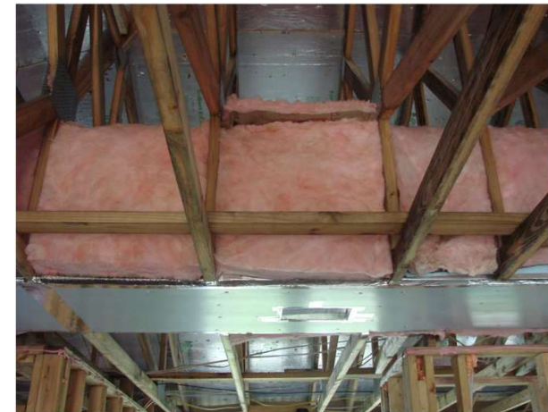
Figure MS-28-b Finished raised ceiling duct chase
