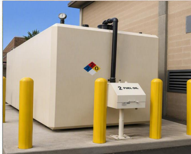
4. Temp. fuel oil storage tank with a capacity \leq 5,000 gal. at a site for emergency use, connected to an exist. oil-burning appliance.
