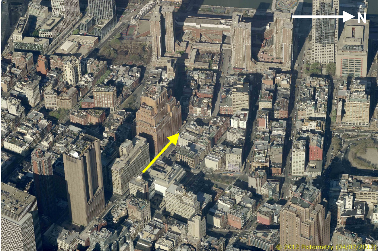
Figure 2 – Project site, with approximate location of the crane at the time of collapse shown by the yellow arrow. The arrow’s direction indicates the viewpoint in Figure 3.
