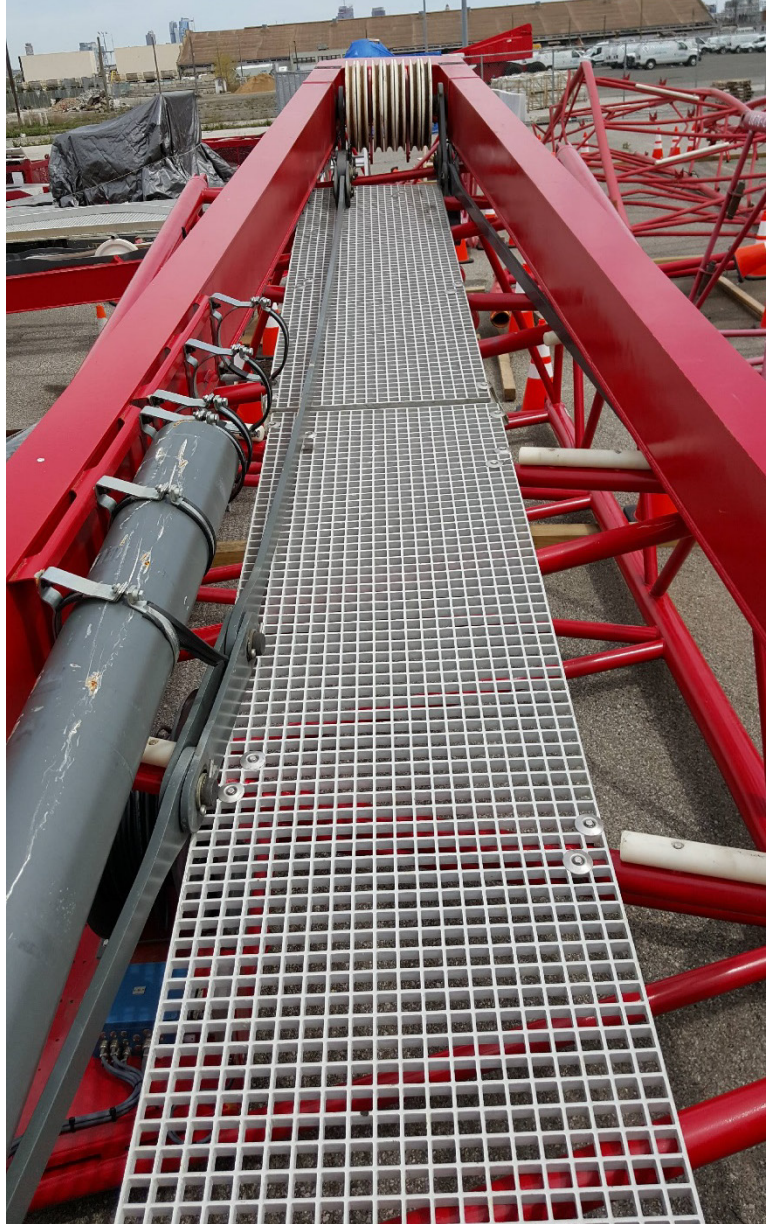
Photo 3 – FRP grating panel fastened to jib heel
