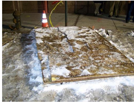
Photograph D.3 (south side)
