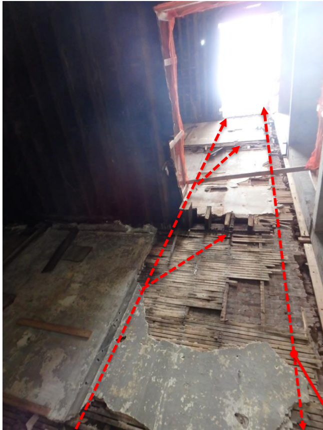
Existing joists cut
