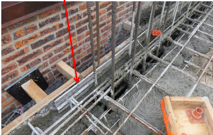
Wet concrete against adjacent existing wall
