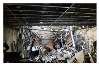
Overloading and improper installation of cold-formed steel including joists, rafters, trusses, and structural wall studs, etc., can result in injury and property damage.
