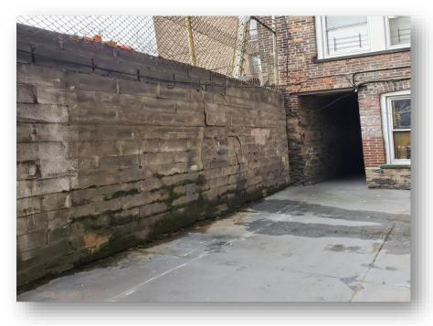
One wall can impact multiple owners, egress pathways, fire escapes, egress corridors. If these areas are blocked due to unsafe or collapsed retaining wall, the building must be vacated until the owner installs fireguards and eventually fixes the wall. Temporary shoring usually blocks these pathways as well.
