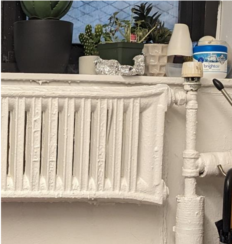
Two-pipe steam radiator with a TRV
