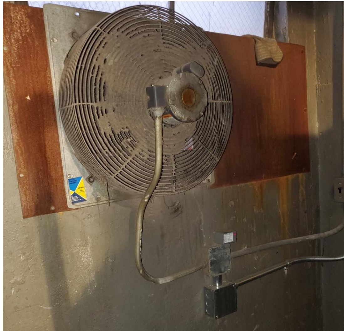
Exhaust fan with timer
