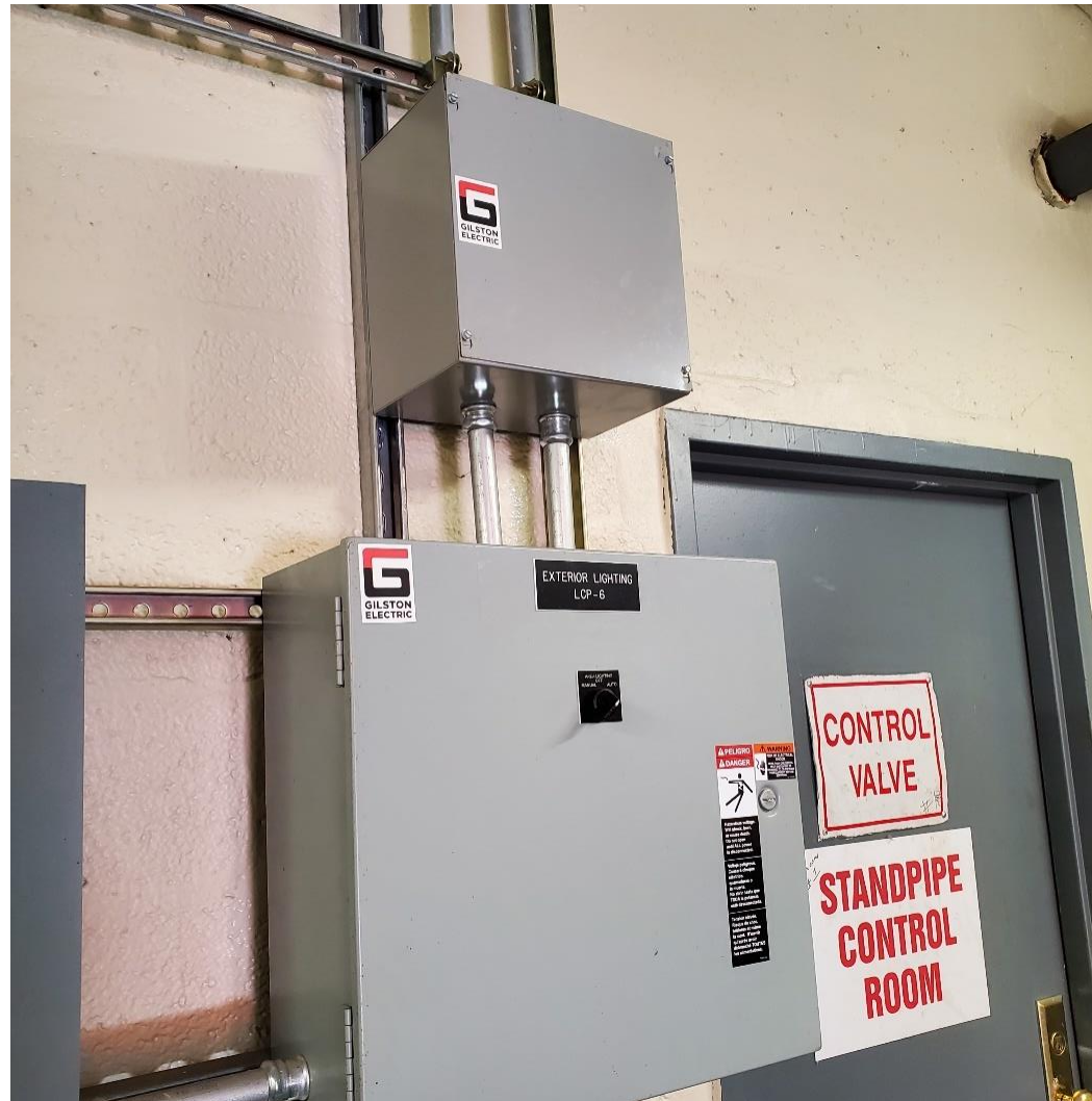
Exterior Lighting Controls
