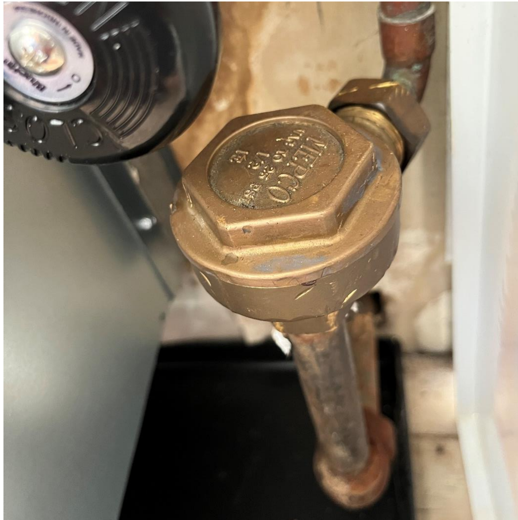
Thermostatic steam trap in a dwelling unit
