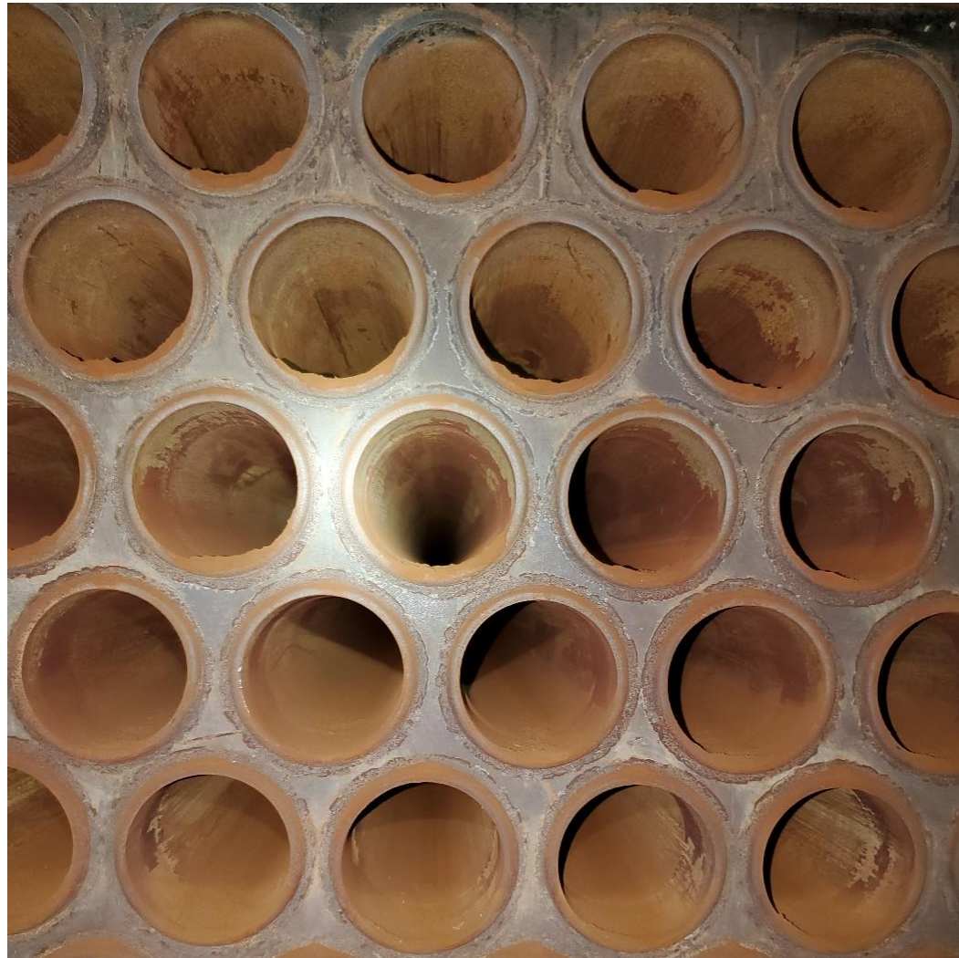
Visual inspection of boiler firetubes
