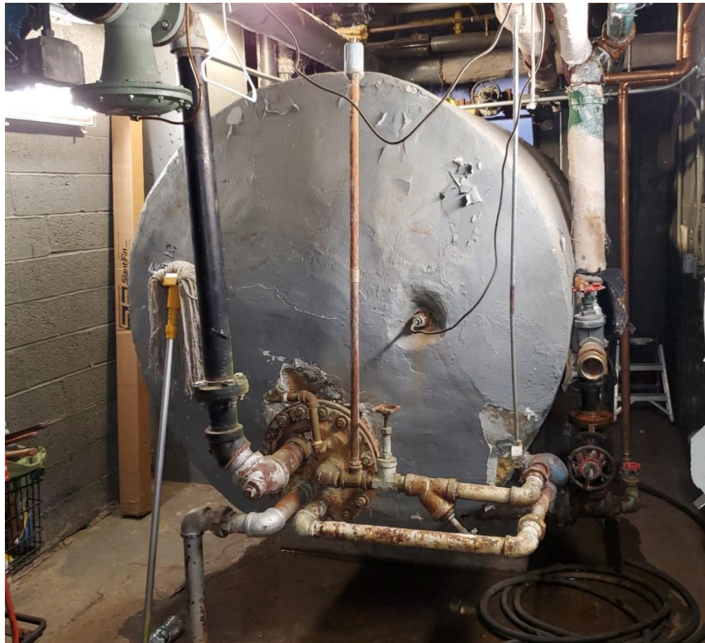
Insulated hot water tank
