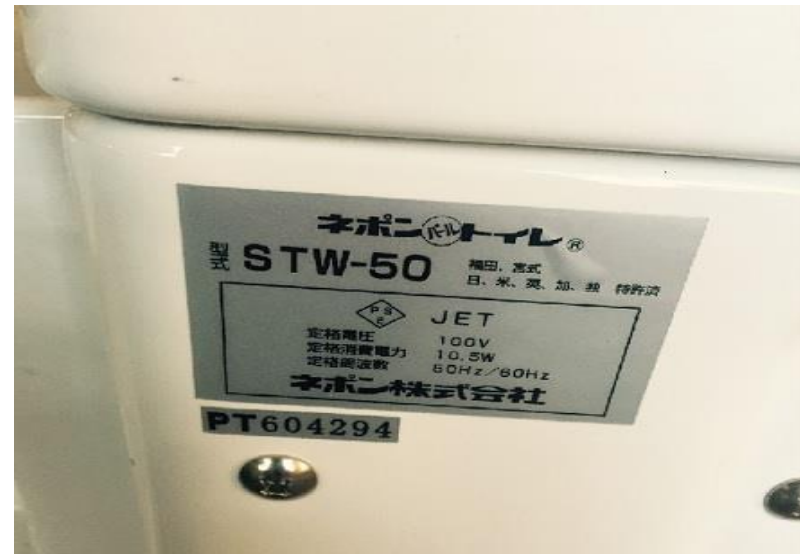
Testing Agency: Japanese Electrical Testing (J.E.T.), not an OSHA recognized testing lab
