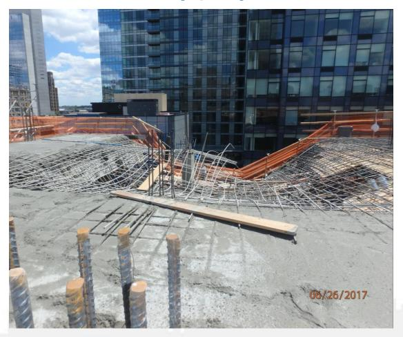
Workers pouring the deck on the 6th floor of the site building shoring posts were not certified and did not meet job specs. The CSM and Formwork designer failed to observe that the shores were undersized and could not support the weight. Six workers were caught in the collapse that caused 12+ yards of concrete to rain down.
