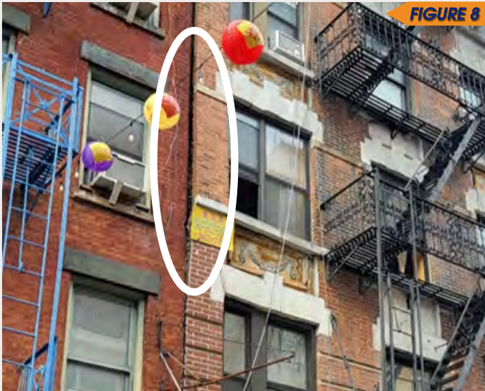
Figures 8 & 9 show exterior façade brick bulged outward.
