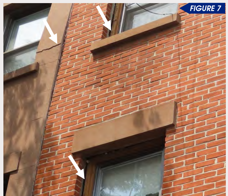
Figures 6 & 7 show bowing of a historic façade wall on typical New York City row houses. Voids are visible in the backup wythes and behind the face brick.
