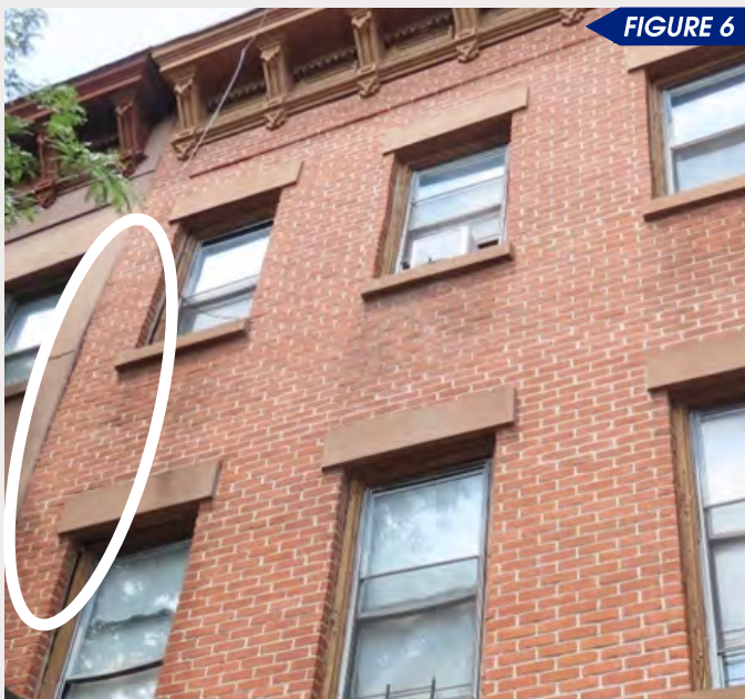
Figures 6 & 7 show bowing of a historic façade wall on typical New York City row houses. Voids are visible in the backup wythes and behind the face brick.
