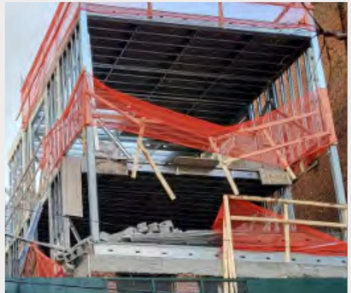
A knuckleboom deposited CMU block on a deck before the framing system was complete, overloading the deck.
