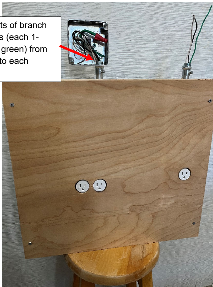
Photo 3 – Installed 22 System Receptacles in Millwork
