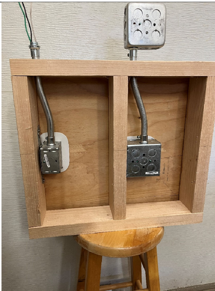
Photo 2 – Mockup Wall Section w/o Surface Rear
