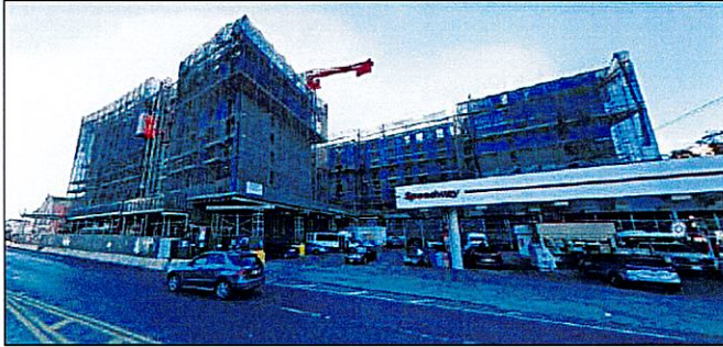
New construction at 548 Utica Ave. just north of the Development Site
