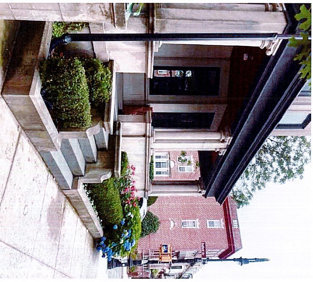
118 Rutland Road – views of repaired stair, curb, & porch Damaged bluestone curb patched & refinished
