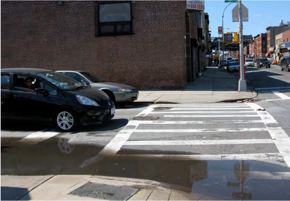
Drainage was identified as an issue in the area even before Hurricane Sandy. Here, significant ponding at the corner of 6th Street and 3rd Avenue in the absence of rain.
