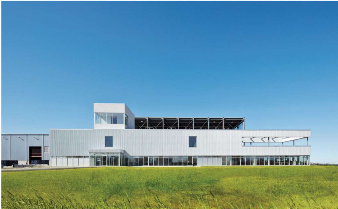
SIMS Municipal Recycling Plant, Sunset Park, Brooklyn, image courtesy of Selldorf Architects
