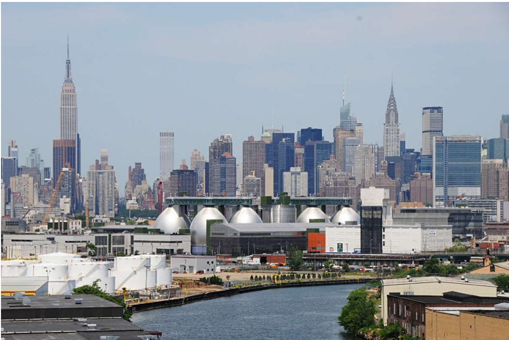
Newtown Creek WWTP, Greenpoint, Brooklyn
