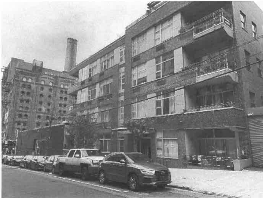
View of the Project Area facing northwest from South 3rd Street.
