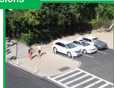
Painted Sidewalk Extensions
