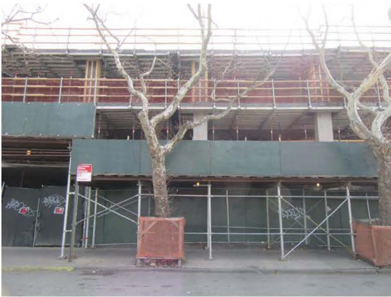
4. View of the Development Site facing southeast from Keap Street.
