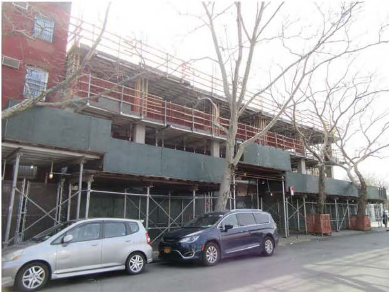
3. View of the Development Site facing south from Keap Street.
